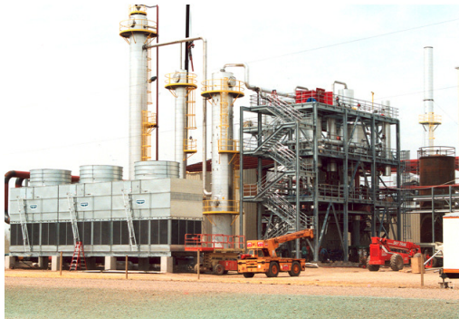
Ace Ethanol Plant, Stanley WI
